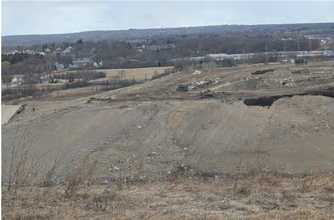
Top of Phase 1 & 2 viewed from South
