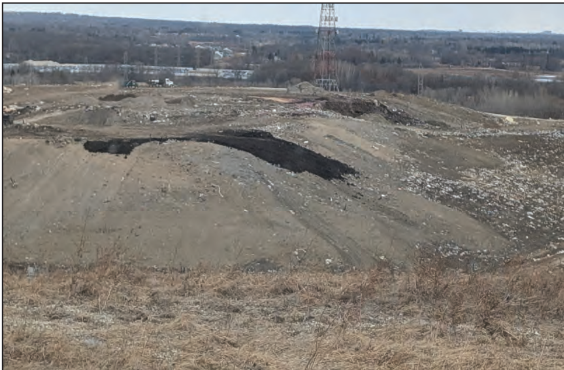
Starting of top soil spread on Phase 1, increases thickness of Intermediate Cover
